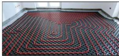
■ Full installation of REHAU VARIONOVA underfloor heating system, ensuring comfort and performance.
